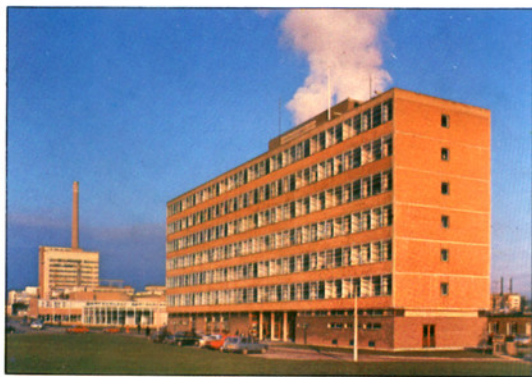
Main administration block, Windscale
