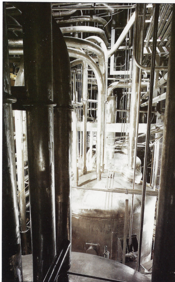
Sea discharge treatment cell vessels and pipework in SIXEP.
