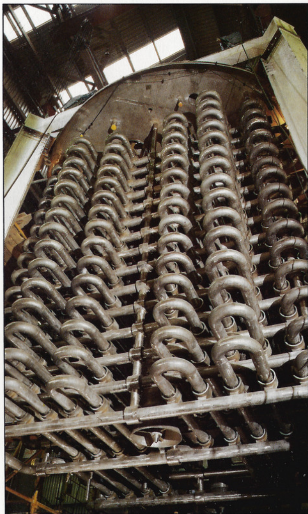
A highly-active waste tank under construction.
