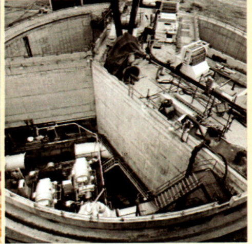
CW Pumphouse and bandscreens in November 1964.
