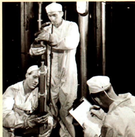
Fuel loading on Reactor One in June 1965.
