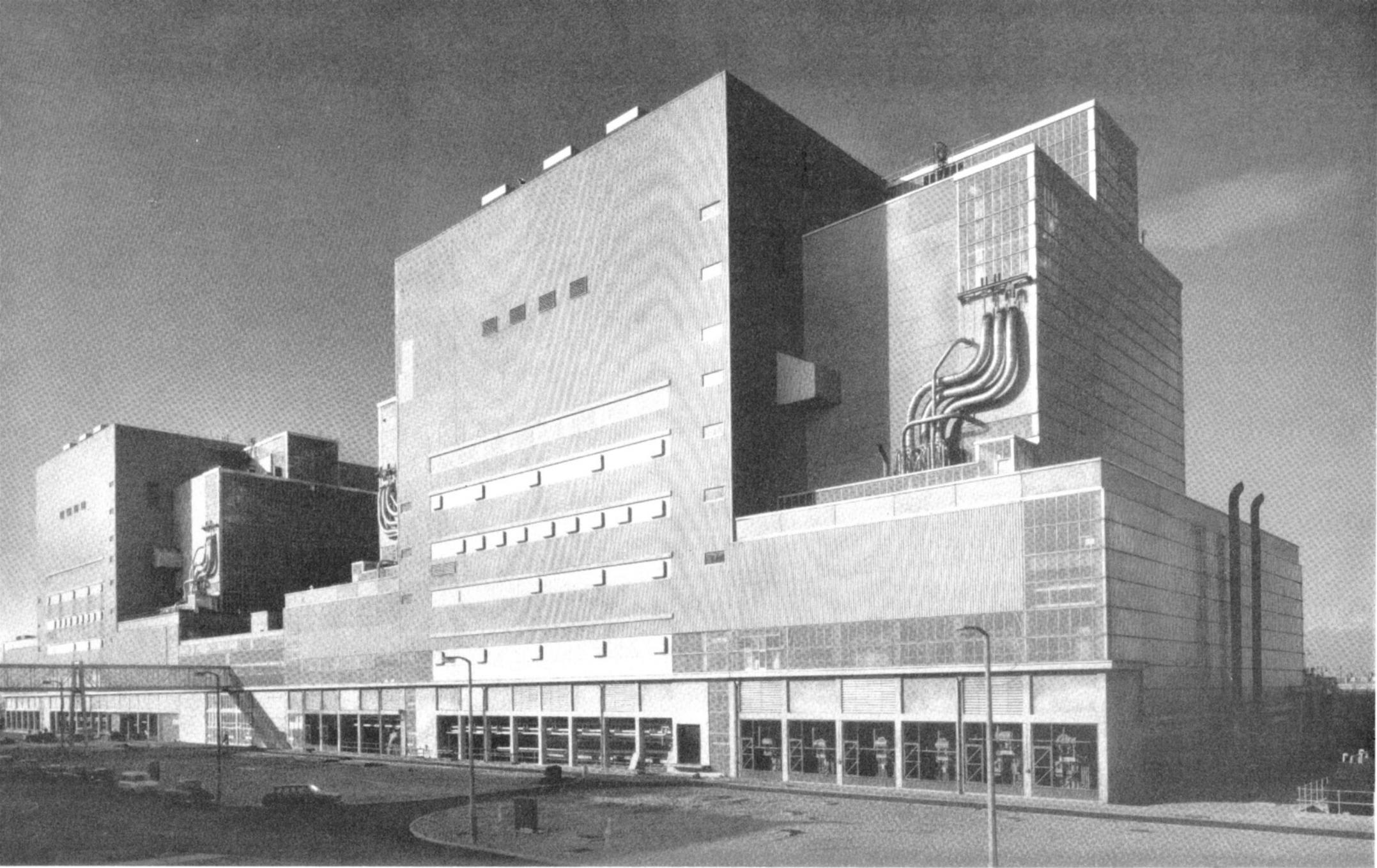
Reactor Buildings from the South East
