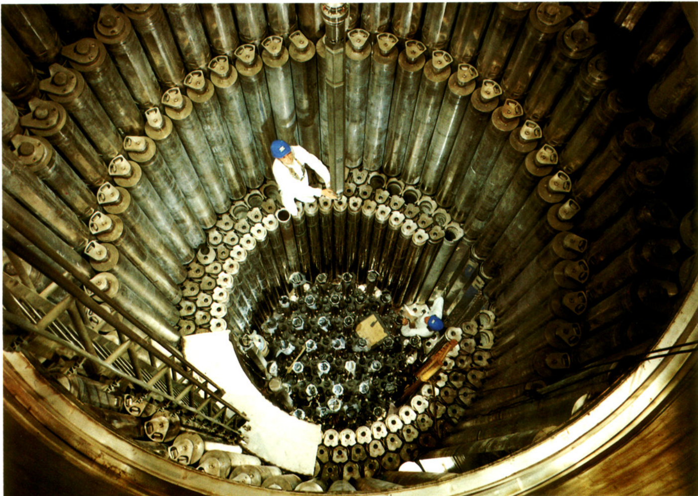
Dummy fuel loading trials in the reactor core during construction.
