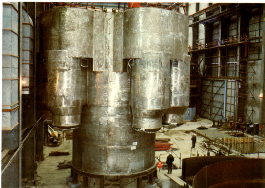
View of the reactor jacket, before suspension in the vault, showing two of the intermediate heat exchanger pods.
