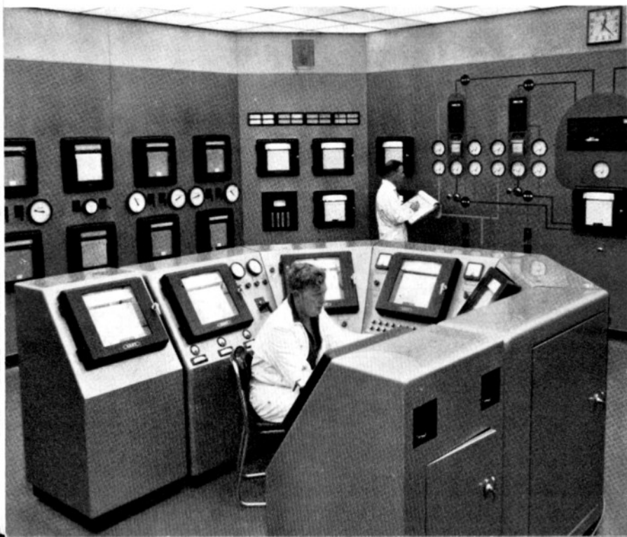
The No. 1 reactor control room at Calder Hall showing the control desk and the instrumentation.
