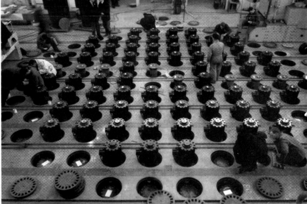
A Reactor Charging Floor.
