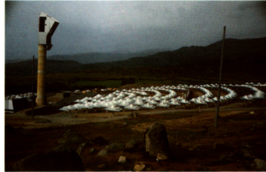
2 MW Themis Solar Power Station, France
