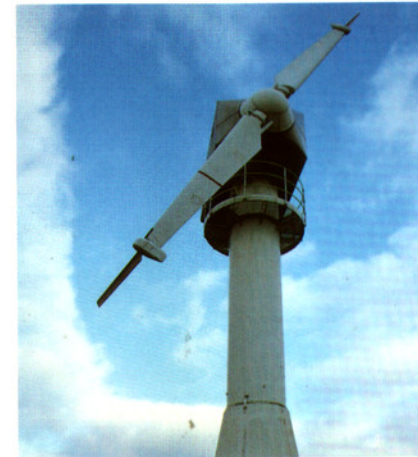
3 MW Wind Turbine generator on Orkney
