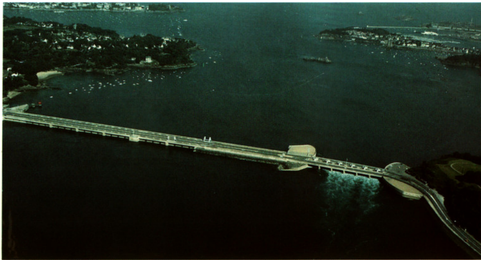
Tidal barrage, Rance Estuary in Brittany, France
