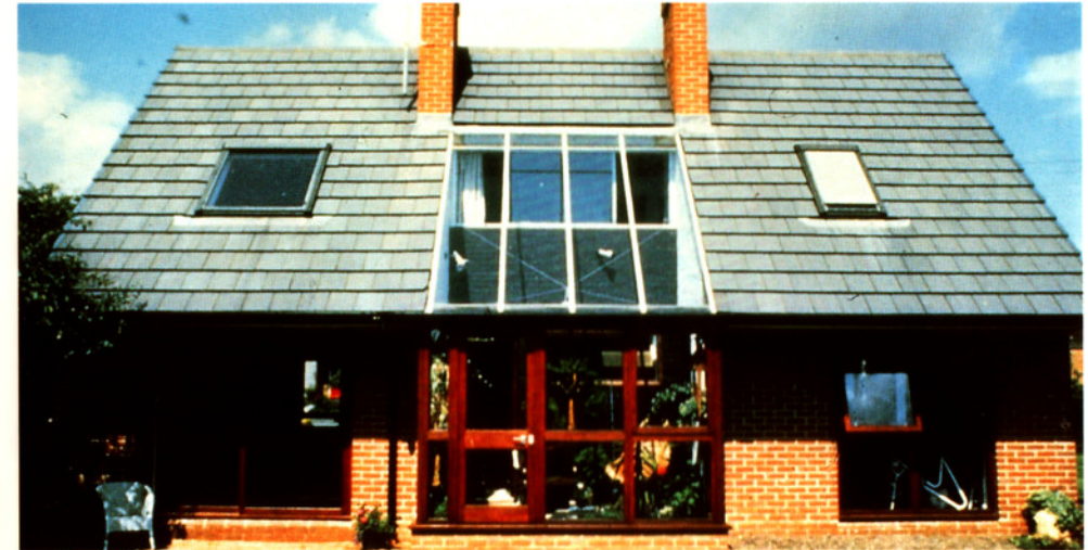
Solar heated building
