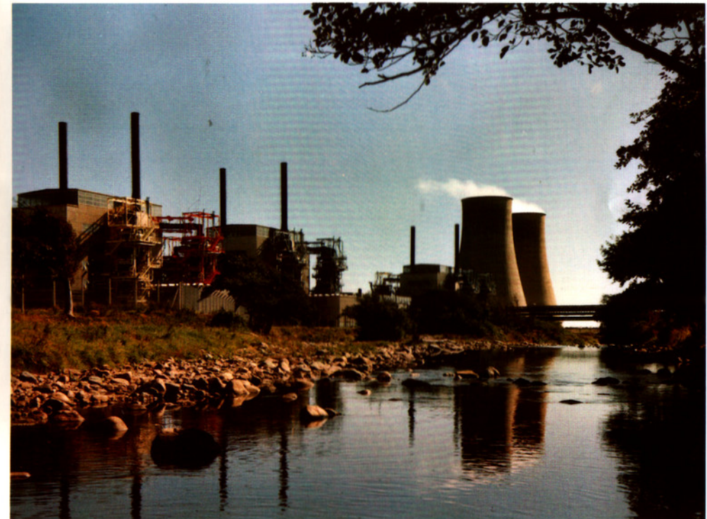
Calder Hall – the world's first nuclear combined heat and power station
